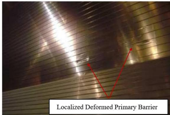
Figure 1-4: Permanent deformation in the primary barrier due to sloshing [21]
