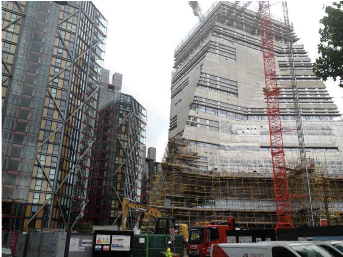
Tate Modern Extension under construction, (2015) Photo: Andrew Dewdney
