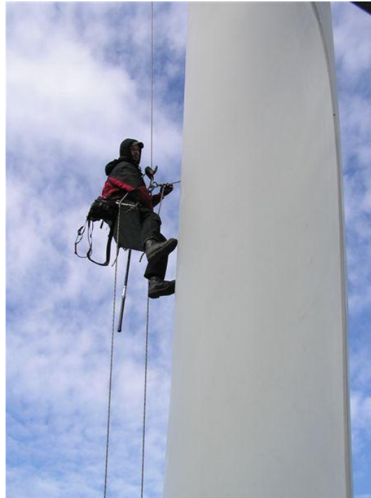
Figure 1.1 Skilled worker climbing a wind turbine blade using ropes hung from the nacelle to inspect the leading and the trailing blade edge [14].
