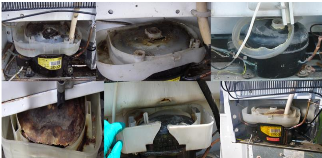
Figure 6.3 Six examples of plastic evaporation trays which have degraded allowing leakage. (Taken from research photos from amenity site visits)
