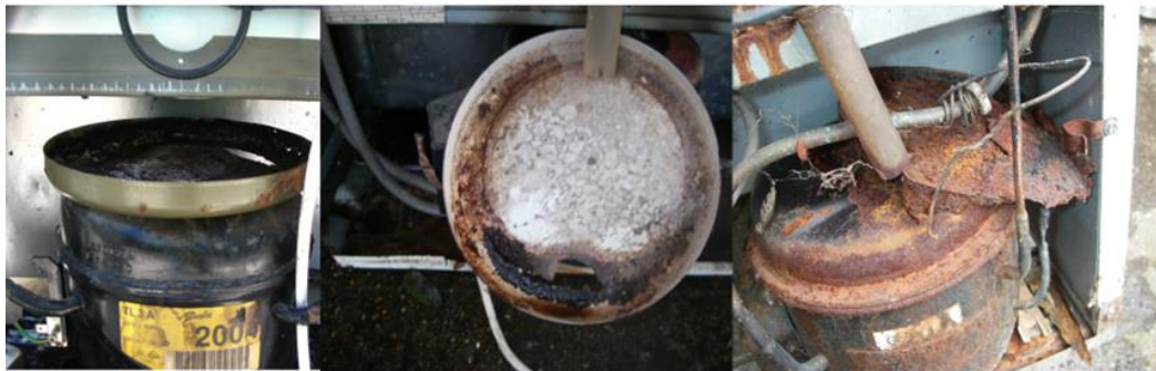
Figure 6.1 Some examples of corroded metal evaporation trays used in older domestic refrigeration appliances.
