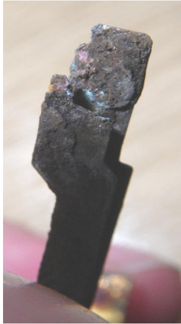
Figure 5.19 An example of the severe arc damage caused to switch contacts.
