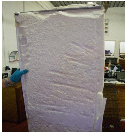
Figure 6-13 Removing the external metal sidewall reveals the hydrocarbon blown polyurethane foam beneath.
