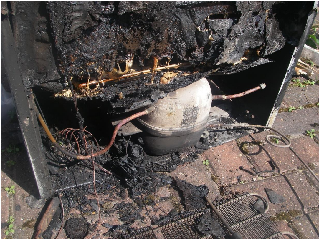
Figure 3.16. Rear of appliance showing low level fire damage and spread through compressor compartment
