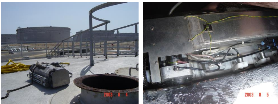
Fig. 6. Left: RobTank before entry through manhole in the roof of a ATG storage tank, Sines oil refinery, Portugal; Right: Ultrasonic NDT tests in oil sludge.
