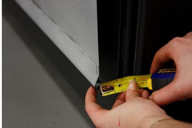
Figure 118. Measuring shading fabric distance
