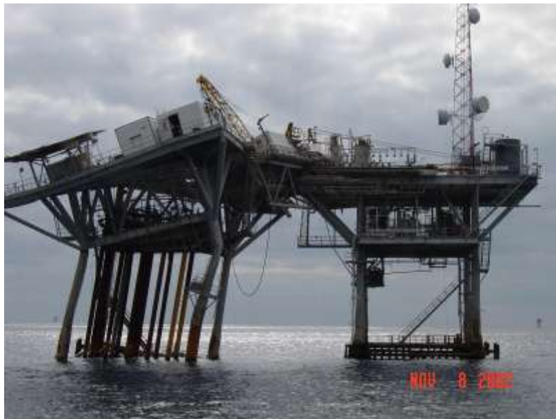
Figure 8.1 Global Structural Failure from Hurricane Lilli (De Franco, 2004)
