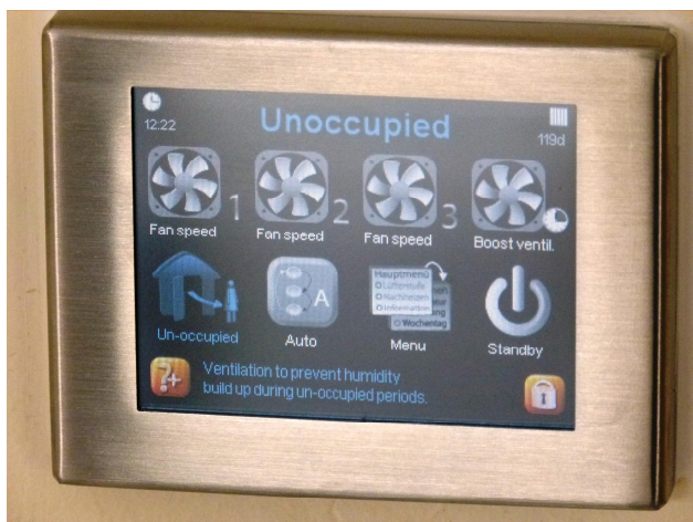
Figure 2 MVHR controls (picture courtesy of Martin Ingham)
