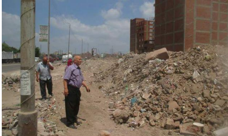
Figure 4. 300 Tonnes of CDW Dumped on Main Roads of Mansoura City
