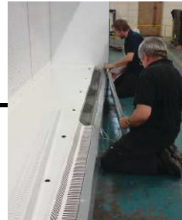
Cabinet is re-assembled with new and remanufactured parts
