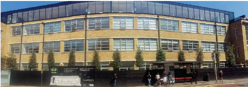
Figure 1. South-West facing building close to Camden High Street Underground Station
