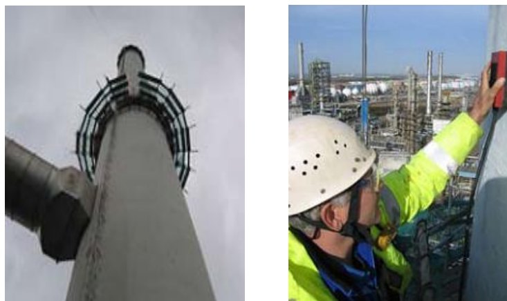
Figure 1-1. Manual NDT of tall concrete cooling tower by erecting scaffolding [7].
