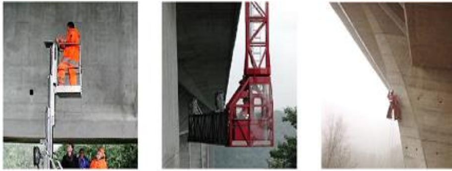
Figure 1-2. Access devices used for vertical structure inspection [8].
