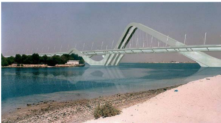
Fig. 3: Sheik Zayed Bridge in Abu Dhabi [23].
