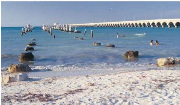
Fig. 1: The Progresso Pier in Mexico [21].
