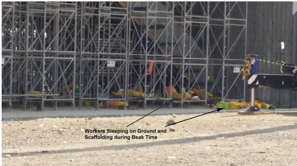
Figure 6: Workers Taking Rest During Break Time on Ground and Scaffolding.
