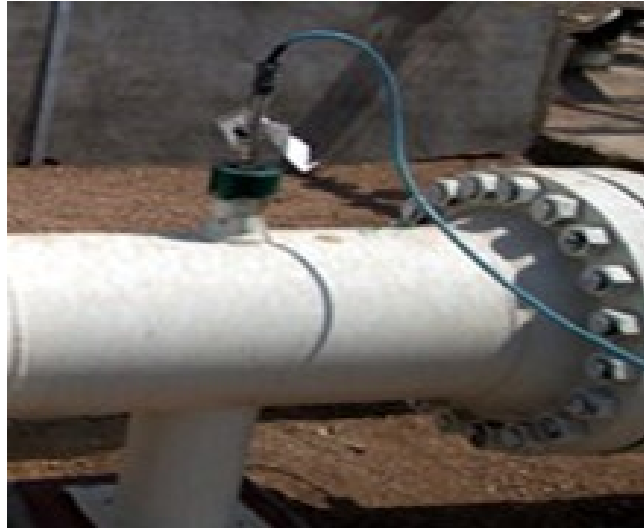
FIGURE 2.1: The installation system for weight loss coupons on pipeline [36].
