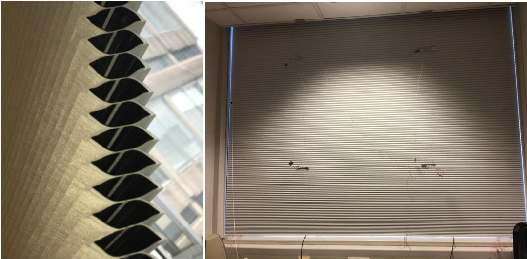
Figure 3: Cellular dimout blind. Left: cellular structure of the blind. Right: representing the blind when it is sealed using side channels
