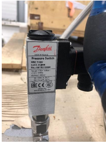
Figure 3. 19 Pressure switches.
