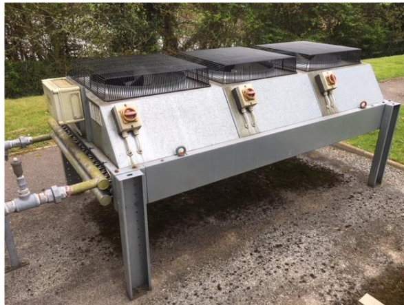
Figure 3.15 Finned-tube water cooler.
