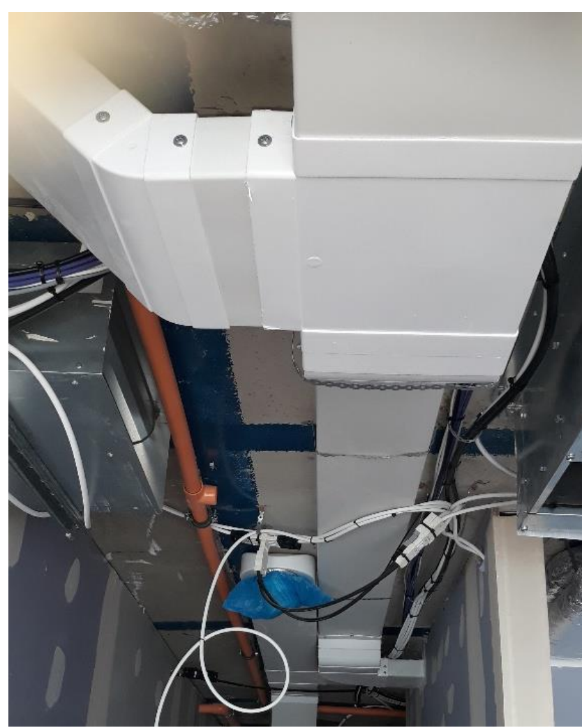
Fig 2. Typical plastic duct T-Branch
