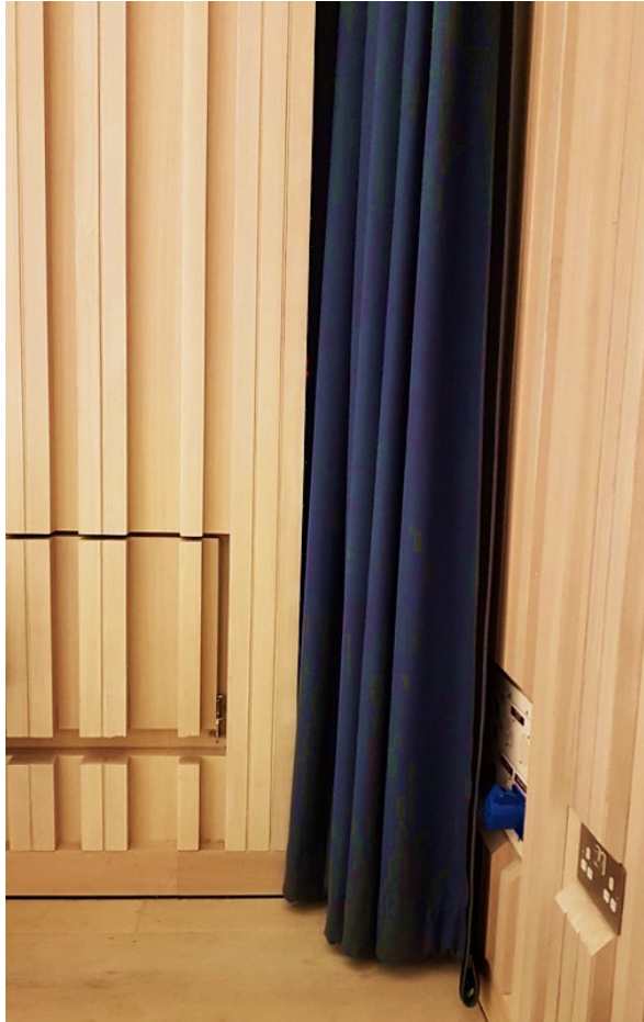
Figure 25: Curtains emerging from their storage position behind the false wall.
