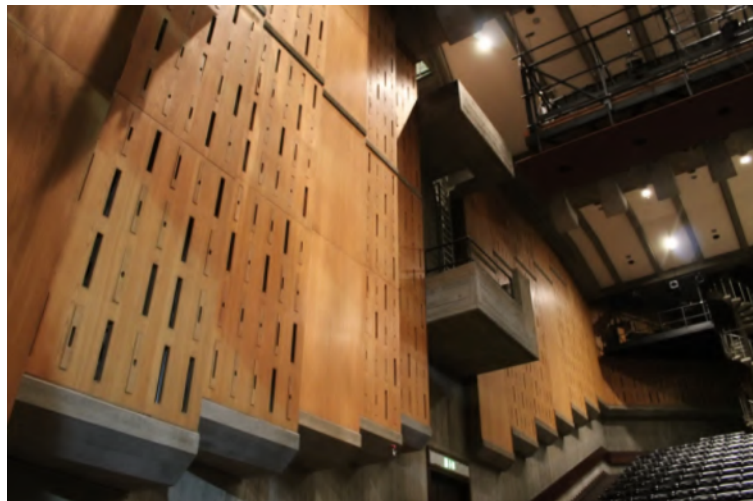
Figure 101: Arrays of Helmholtz resonators lining the side walls of the Queen Elizabeth Hall in London [177].
