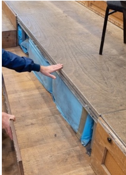
Figure 59: The plastic-wrapped porous absorber underneath the rostra in Henry Wood Hall.
