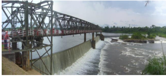
Figure 2.22 Edea power station Source Eneo/AS Sonel (2015)
