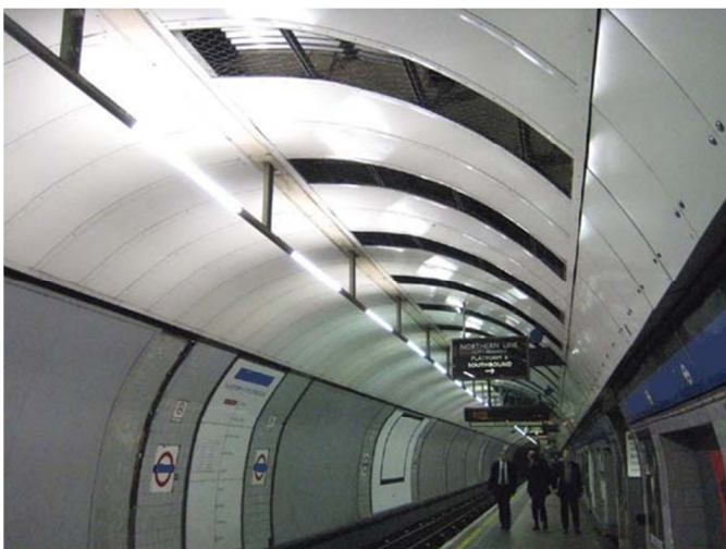
Figure 7:23 Current platform ceiling metal cladding
