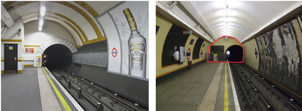
Figure 7:22 Deep platform end walls; marked in red is the virtual open end if high sound absorbency is applied to the end wall
