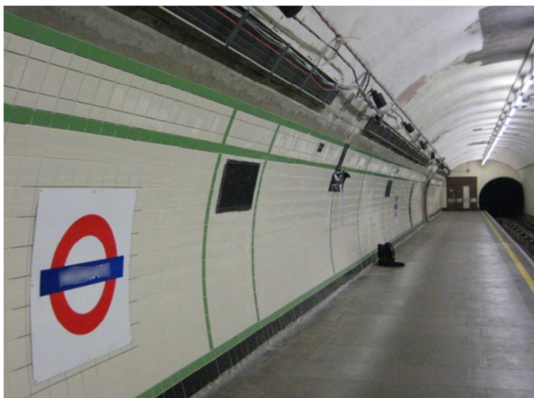
Figure 7:6 Platform during maintenance works showing CMS and projector on wall configuration.
