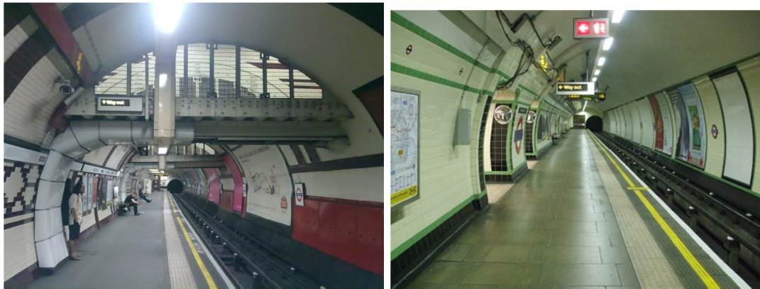
Figure 5:3 Left: platform with over bridges of acoustically transparent sides; Right: platform showing two central wide cross-passages.
