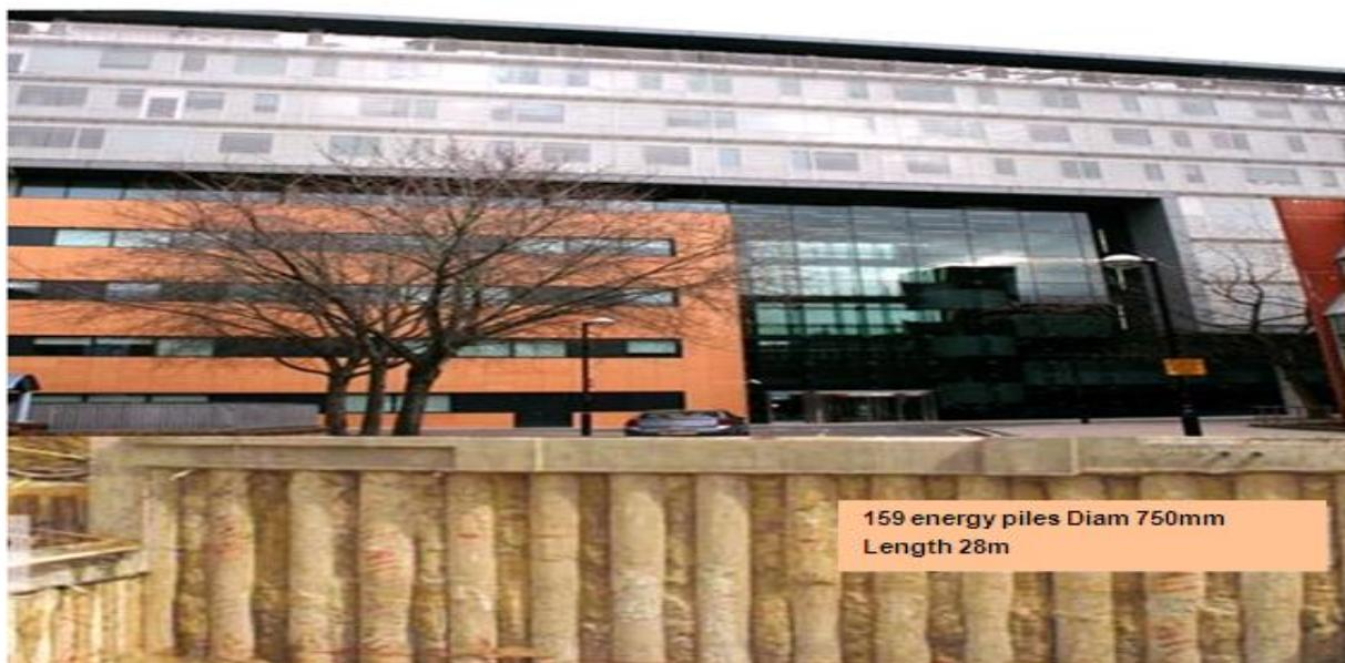
**Figure 4.16** K2 building with its thermopile foundation
