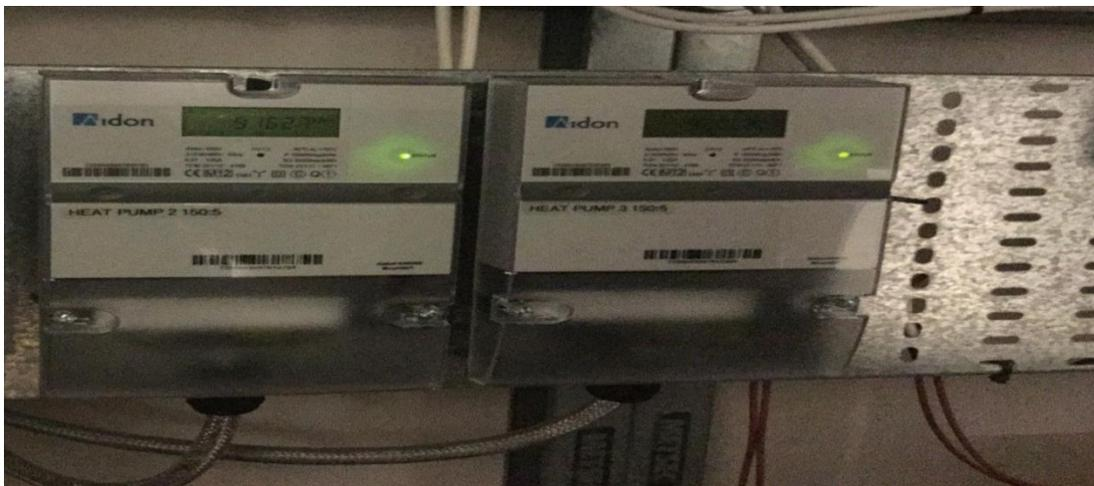
**Figure 4.25** *Aidon 6000-series electricity meter*
