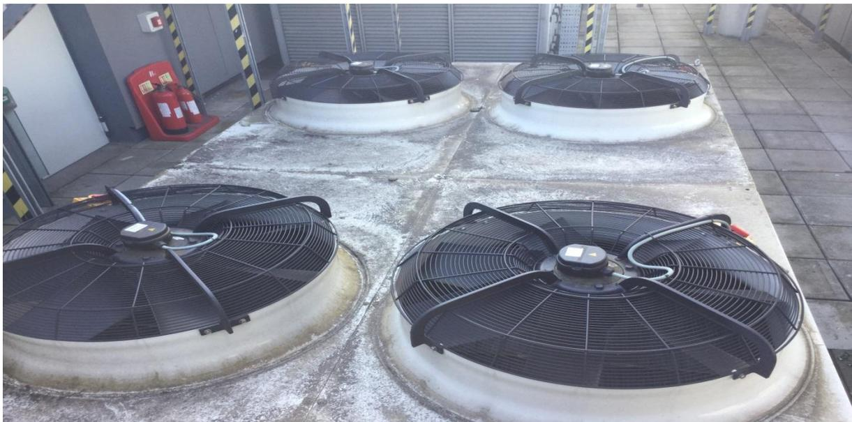
**Figure 4.20** *Dry Air Cooler AlfaBlue BDDT902D*
