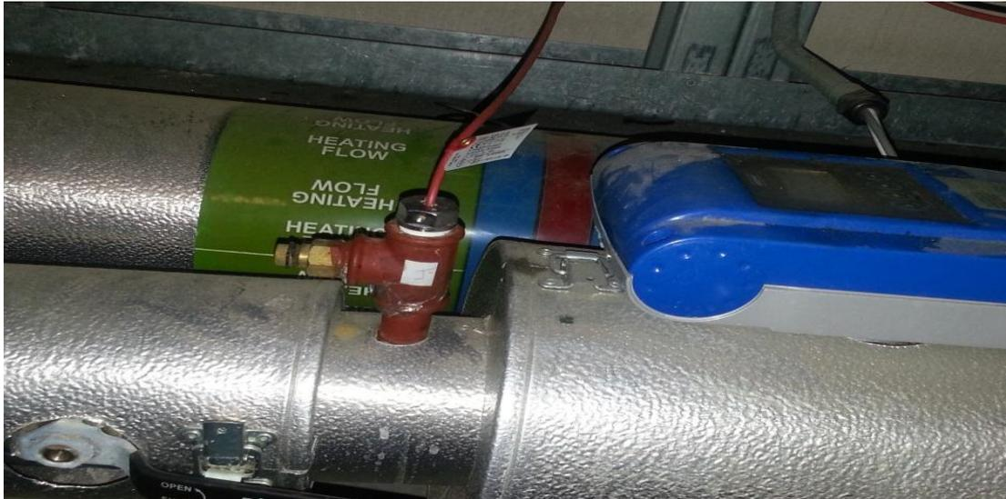
**Figure 4.24** *Krohne OPTIFLUX 4100 Electromagnetic Flowmeter*
