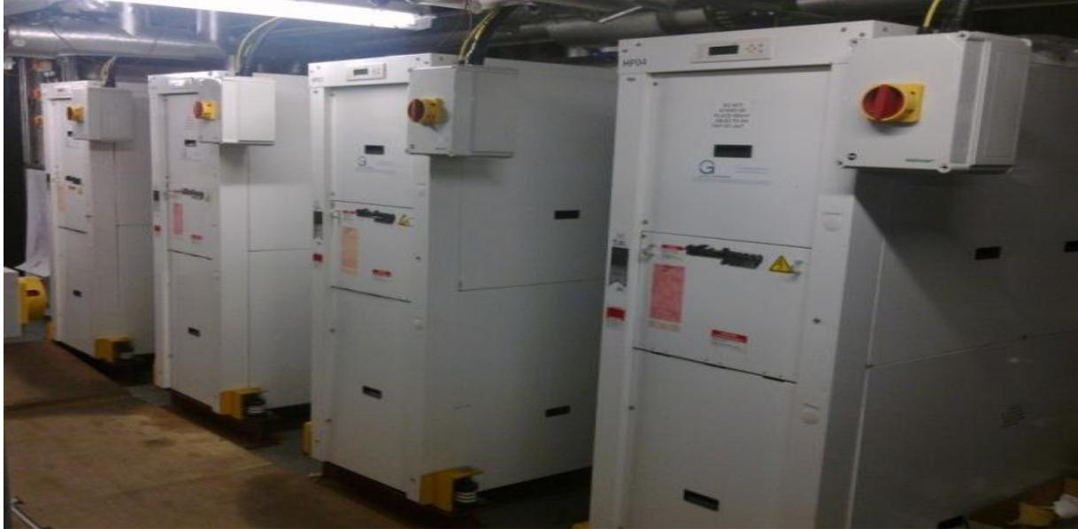
**Figure 4.18** Four WaterFurnace EKW130 HPs installed at K2
