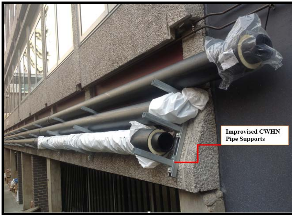
Figure 4 – CWHN pipe work installation
