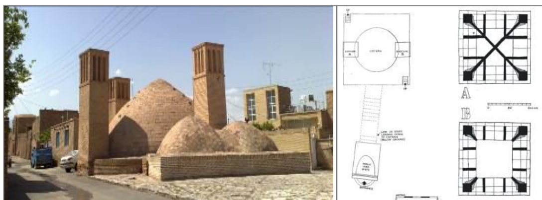
Figure 19: Cistern roof plan and wind catcher detailed plans (Right)
