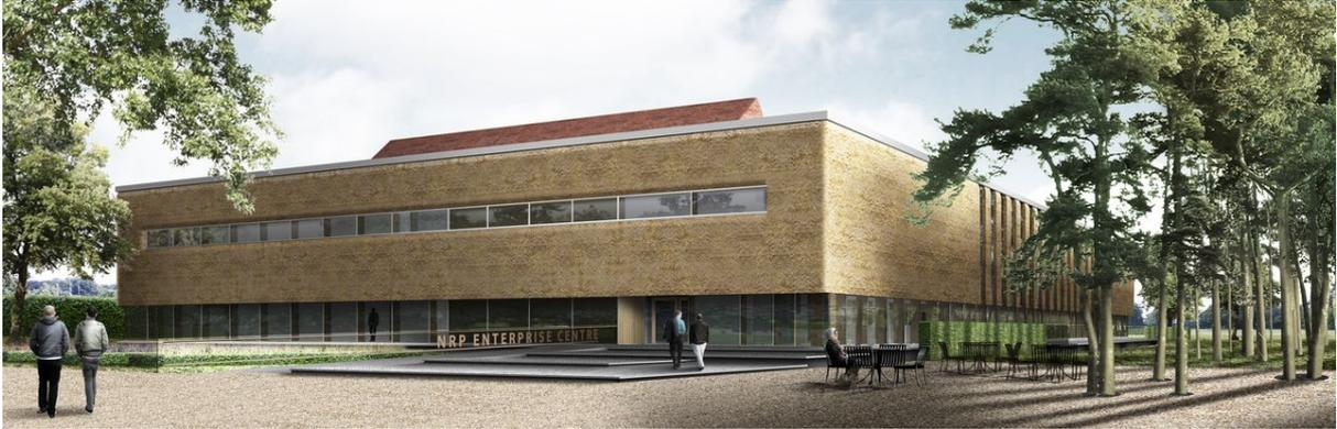
The building is designed to be constructed from a hybrid glulam, Brettstapel and Larsen truss structure, using local timber acquired from the East Anglian region (such as Thetford forest); a rammed chalk lecture theatre; and East Anglian grown hemp insulation throughout. The use of these local materials is to promote activity in the regional timber supply chain and decrease life cycle carbon emissions.
