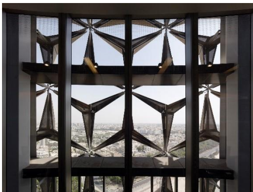
Figure 37 The view from inside to the outside of the Al-Bahr towers (Al Bahr Towers, 2011)
