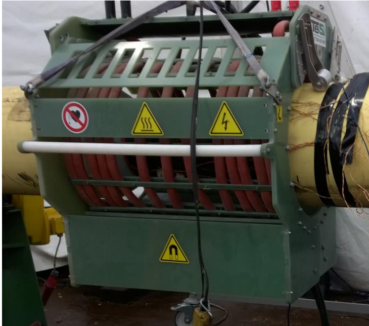
Figure 6: Induction heater installed around field joint.
