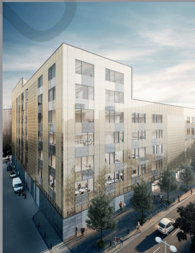
► Figure 3.15 Urban Sciences Building, University of Newcastle
