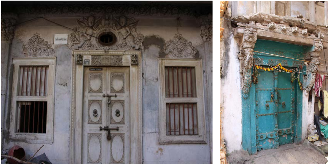
Figure 12 & 13: Door and window design and decoration of heritage houses (Gopipura)
