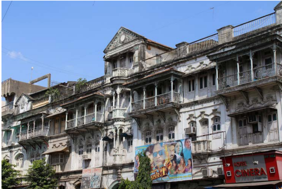
Figure 10: Façade elements with Art Deco influence (Cinema road)
