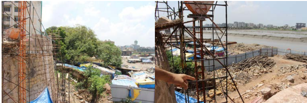
Figure 19 & 20: Restoration of Surat Fort wall along the river edge
