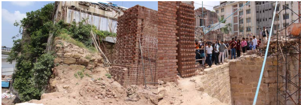
Figure 21 & 22: Redevelopment occurring alongside the old Surat fort walls
