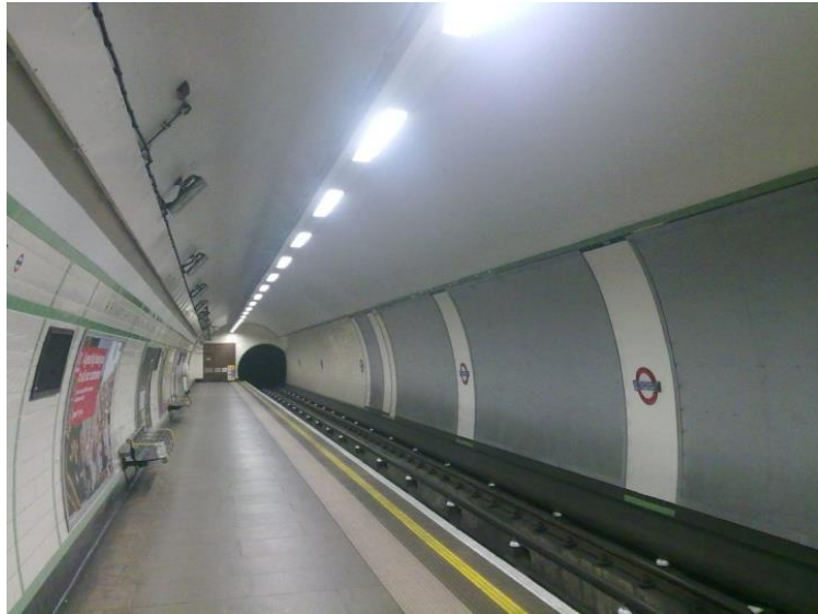
Figure 5 Typical London underground deep platform
