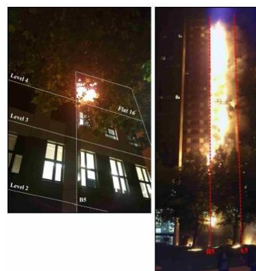
Figure 2: The origin of the fire in Flat 16, 4 th floor + fast vertical spread of the flames
