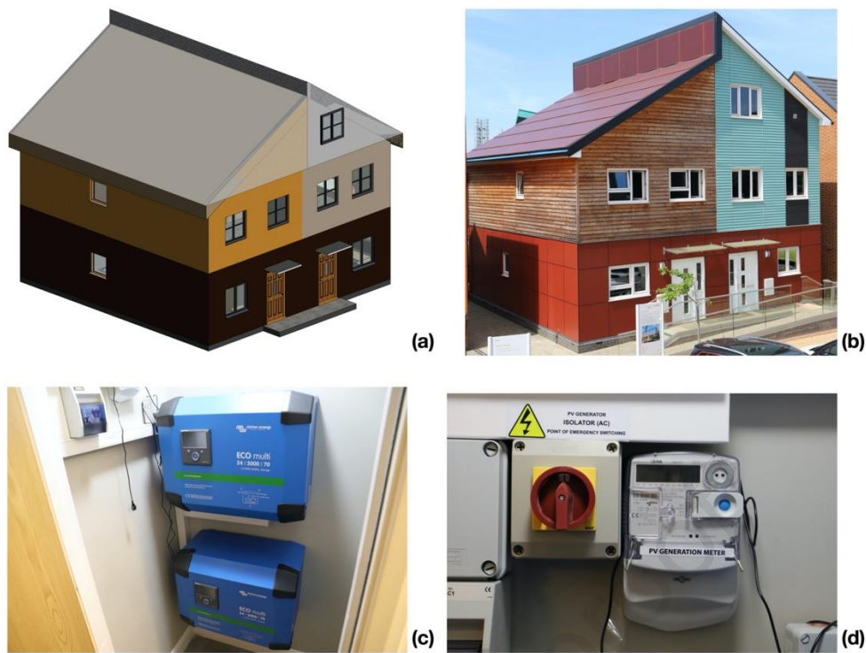
Fig. 4. (a) 3D rendering model of the prototype case study building. (b) The integration of terra-cotta photovoltaic panel systems on the south facing inclined roof surface. (c) The installation of energy batteries into the battery room which is located beneath the staircases in the case study building. (d) The installation of the photovoltaic generation meter to monitor the renewable energy stored.
