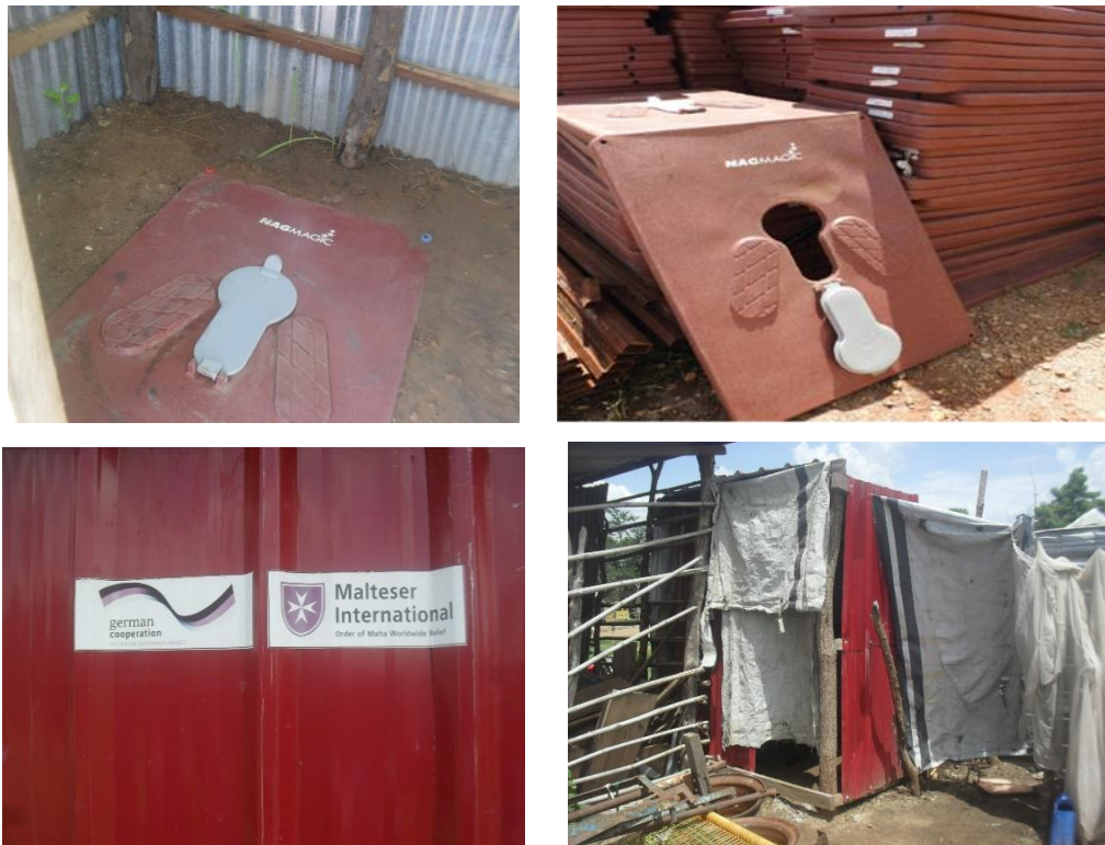
A plastic slab in a pit latrine in Gumbo; Plastic slab at an IOM warehouse in preparation for distribution; Malteser International logo on an iron sheet for latrine superstructure; A latrine with Malteser International latrine materials nearing completion.
