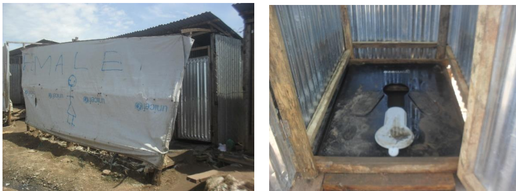
Privacy screen in front of a female latrine block in PoC Site 1; Latrine pit upgraded to concrete from iron sheet.
