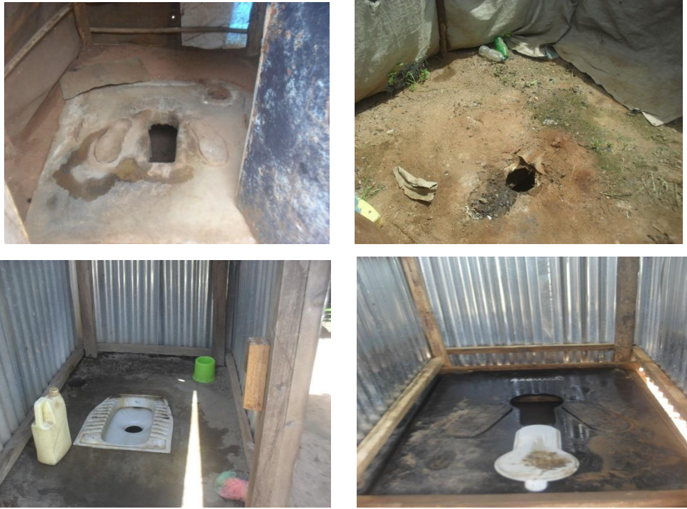
Clockwise: A pre-cast concrete slab; A latrine with no slab; A concrete slab; A plastic slab.
