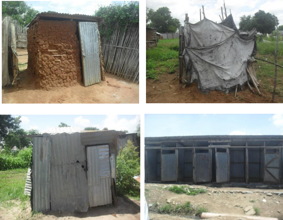
Clockwise: Traditional pit latrine made of mud and bamboo in Gumbo; Simple pit latrine with sack and bamboo superstructure in Lologo; Communal trench latrine block in POC Site 1.
