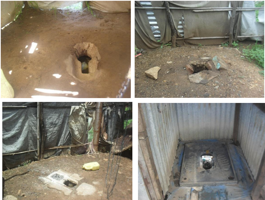
Clockwise: A full pit latrine in Gumbo; A pit latrine with wide drop hole in Lologo; A pit latrine with limited privacy in Lologo; A stance of one of the communal trench latrines in PoC Site 1 with open rear pit and faeces on it.
