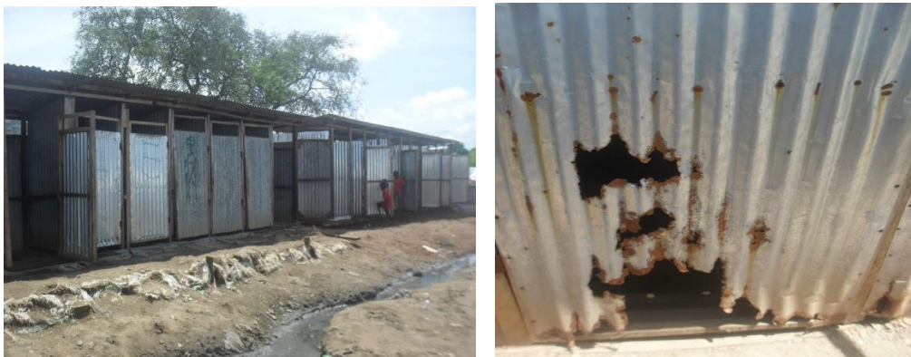
Male and female latrine blocks situated beside each other; Rusting latrine door.
