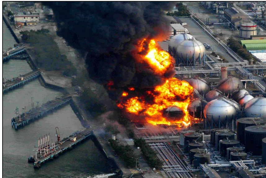
Figure 1-4: Hydrogen explosions at the Fukushima Daichaii nuclear power plant [Opensourceinvestigations.com]
