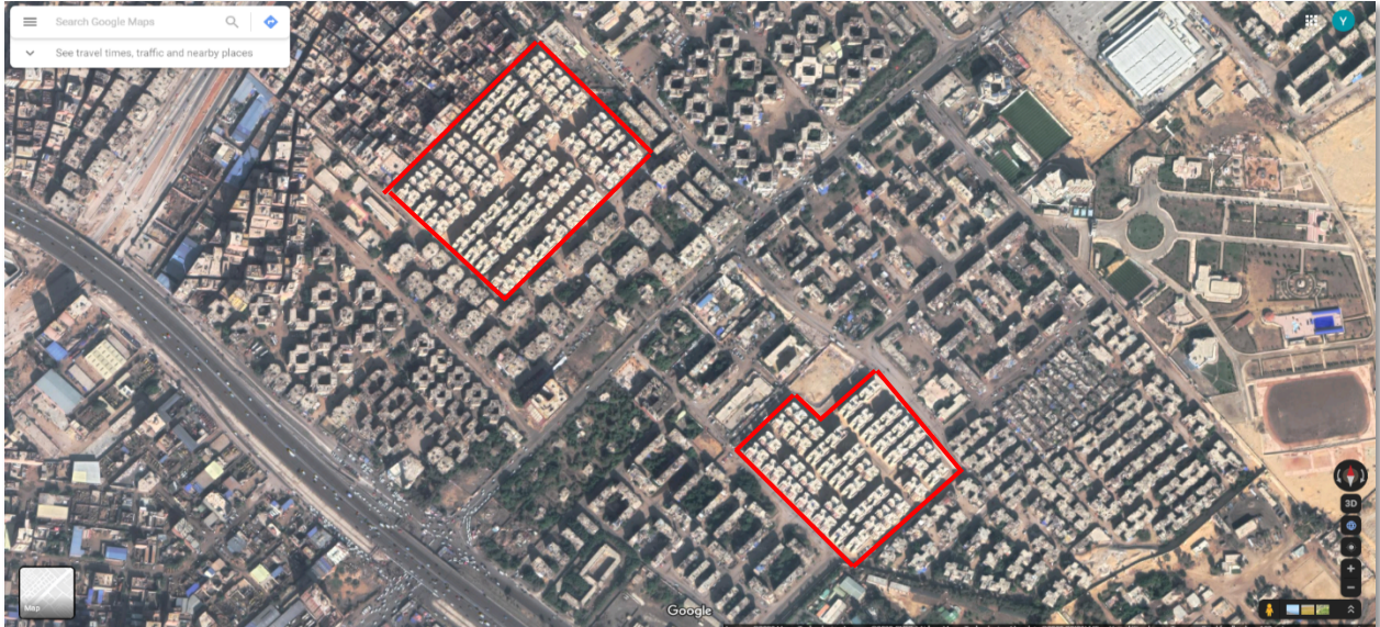
Figure 4.4: Aerial view of Cairo Project CS1 (Google maps, 2020)
