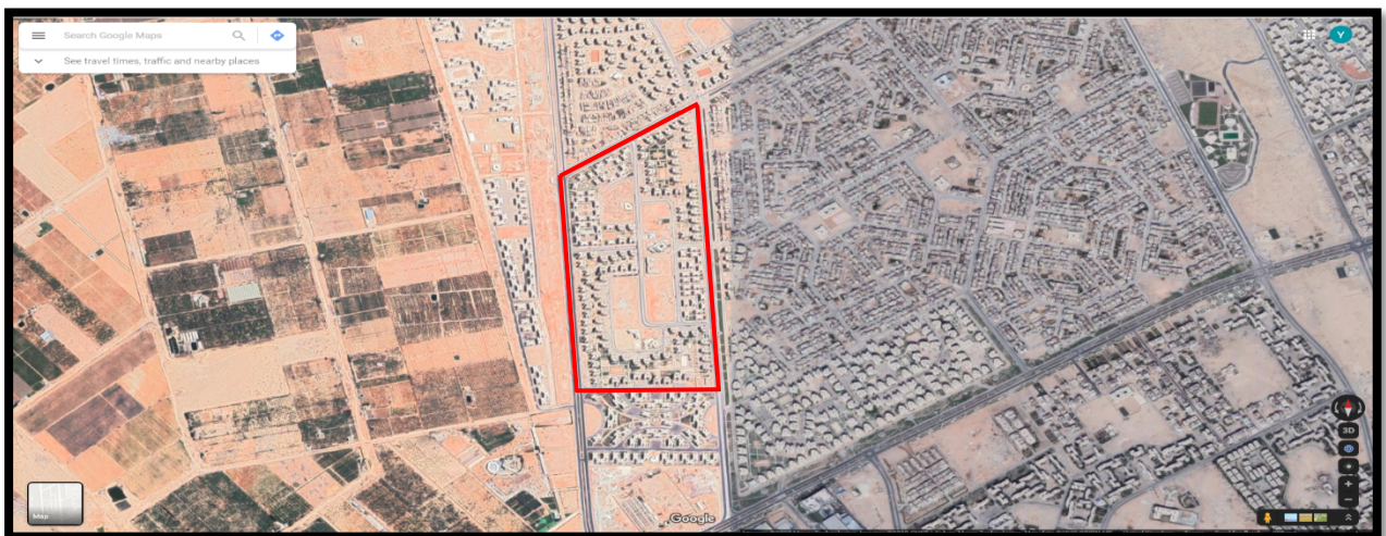
Figure 4.5: Aerial View of Ash Sharqia Project (CS2) (Google maps, 2020)
