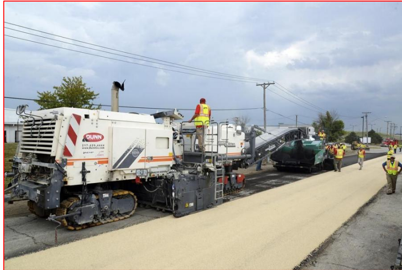
Figure 2.22 Cold in-place recycling (Source: Construction Equipment Guide, 2014)
