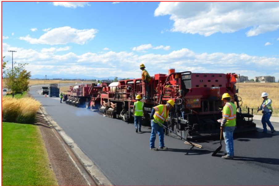
Figure 2.20 Hot mix asphalt recycling (Source: Wells, 2018)
