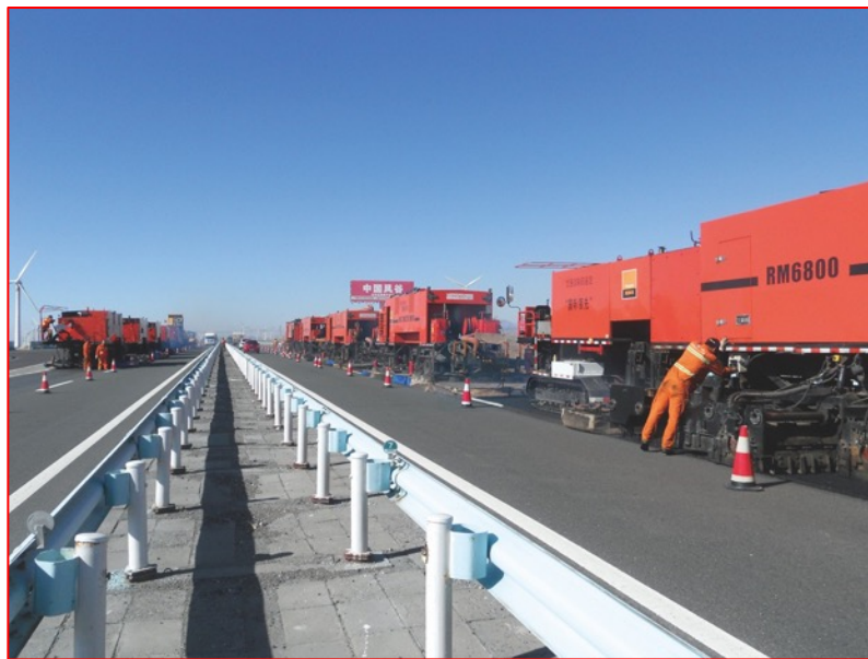
Figure 2.21 Hot in-place recycling (Source: Davis, 2018)
