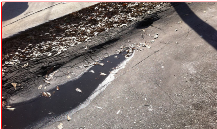
Figure 2.18 Rutting (Source: Neal, 2013)
