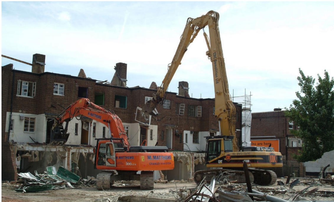
Figure 1.2 Demolition site waste (Source: The Author)
