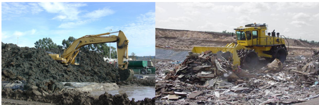
Figure 1.3 Excavation waste (Source: The Author)
