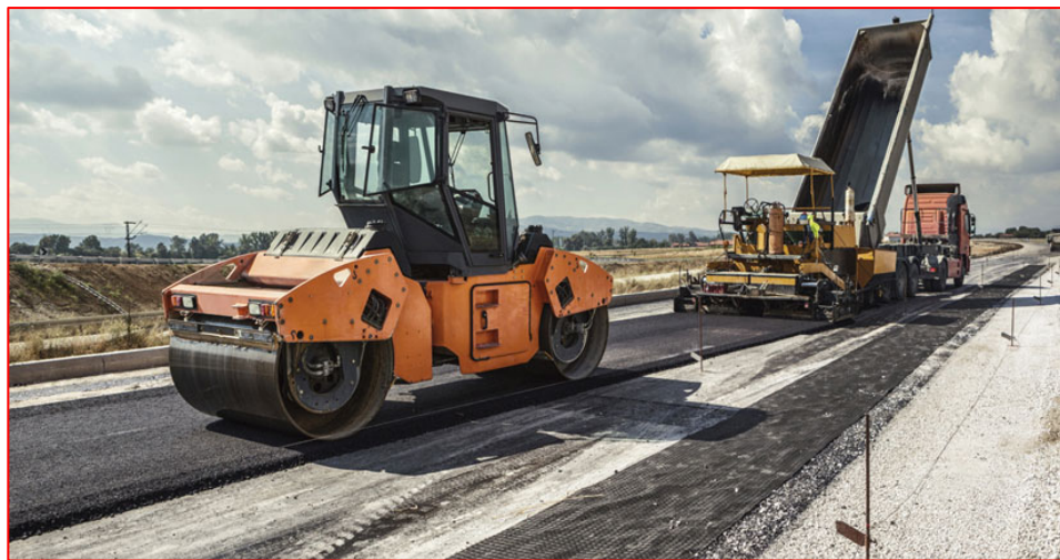
Figure 2.23 Full depth recycling (Source: Mallick & Veeraragavan, 2017)
